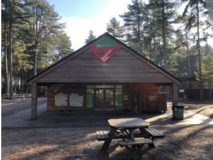
Visitor Centre (Front)
